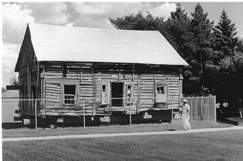
Delorme house (built in 1850s) was moved from River Lot 21 at Pointe Coupée (St. Adolphe) to its present location at St. Norbert Provincial Heritage Park. The house has a post and sill construction known as Red River frame construction.
